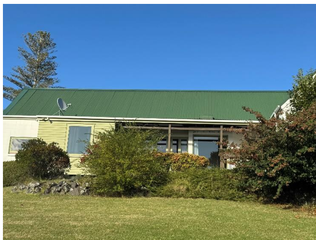
View of vicarage from driveway
